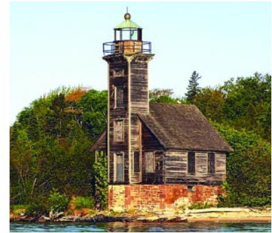
East Channel Lighthouse. Photograph by Dennis O'Hara.
