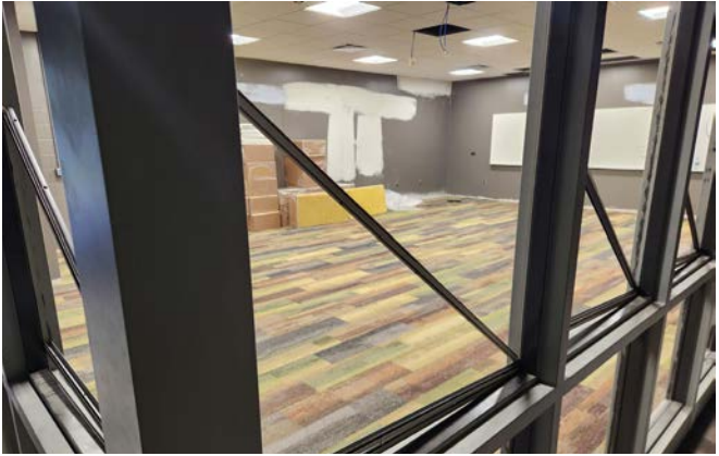
Renovated classroom near HVAC lab
