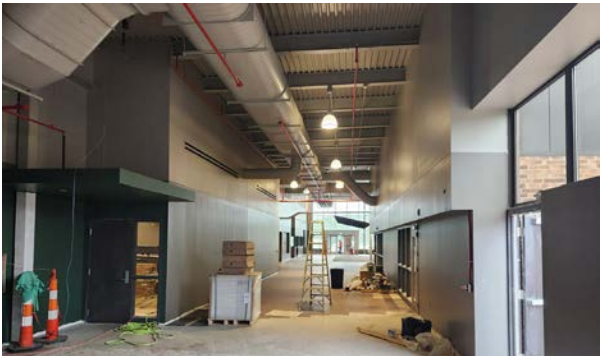
Main corridor looking south
